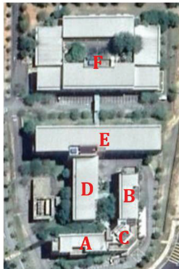
Figure 3: Aerial view of buildings in FKE
